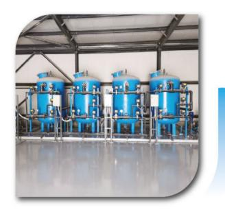
Media filtration is a frequently used process because it is very robust method to remove suspended solids from water.
